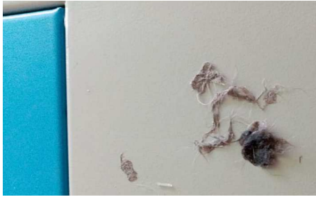
Actual cat hair removed from a tube, pipes and water flow sensor.
